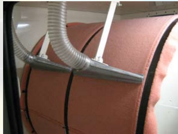
Figure 9 - Zippered Media Installed
