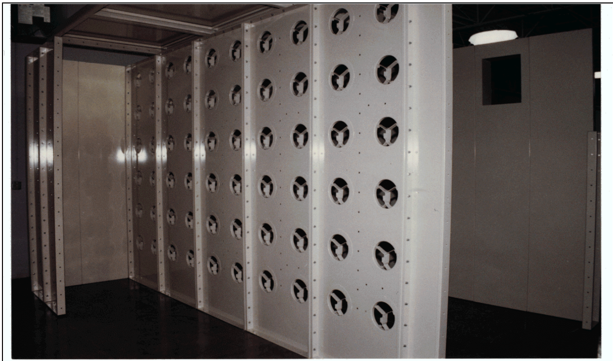
Figure 3 Assembled tube sheet panels and tube sheet flashing from a stand alone Final Filter.
